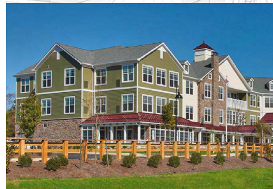
This senior housing example from the northeast, uses varied materials & fenestration to create a neighborhood scale & character
