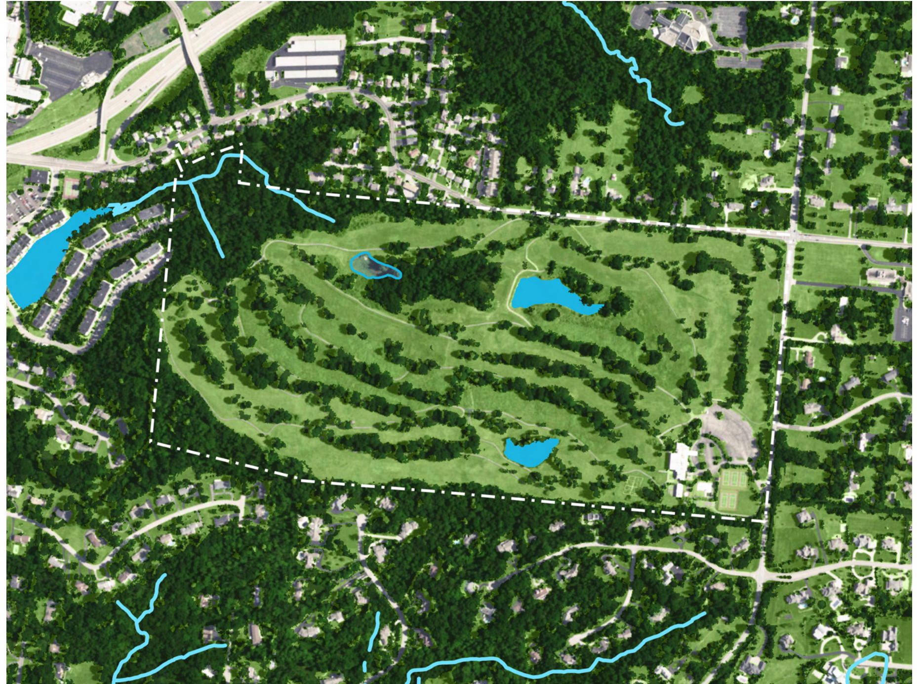
Amberley Green - Existing Conditions
