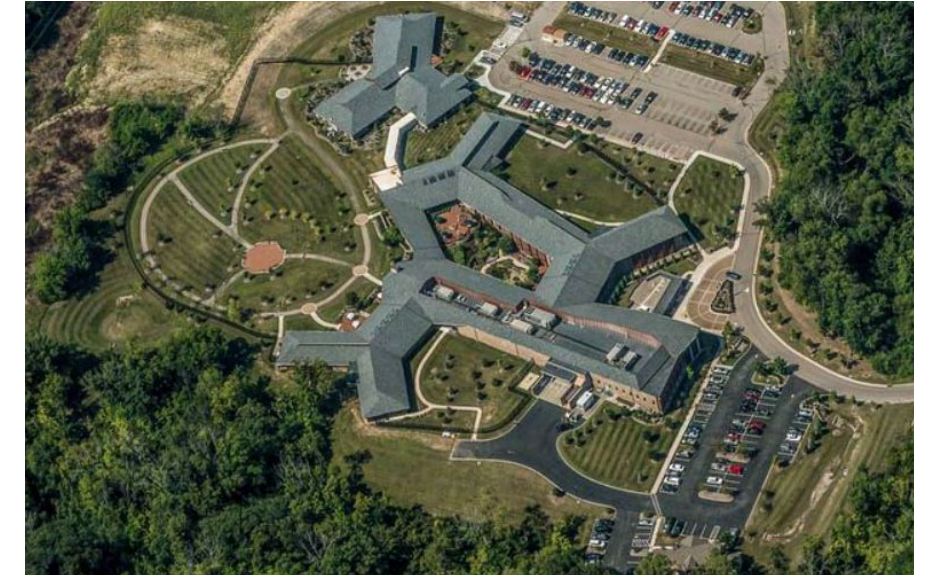
The Lindner Center of Hope could serve as a local precedent for low-impact campus development.
