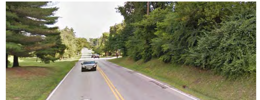
Steep Slope: This condition would likely require a retaining wall to minimize the disturbance along the Right of Way.
