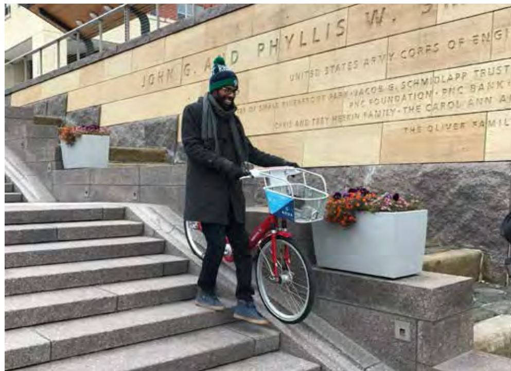
PAVED STAIRS WITH RUNNEL
